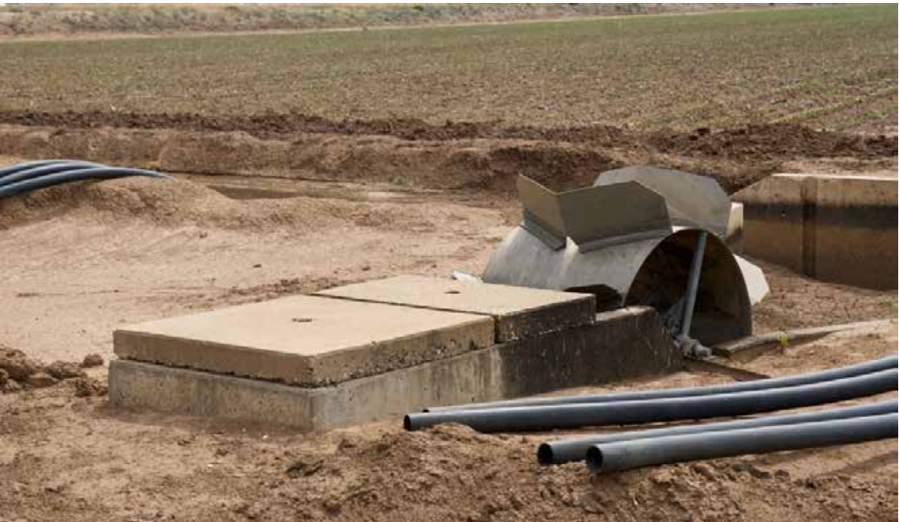
A Dethridge Wheel for metering water flows and siphon tubing for irrigation near St George, Queensland (2008).
